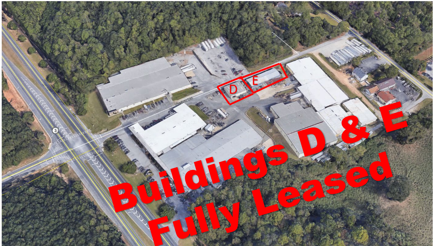
Property Profile – Building D & E (Warehouses)
